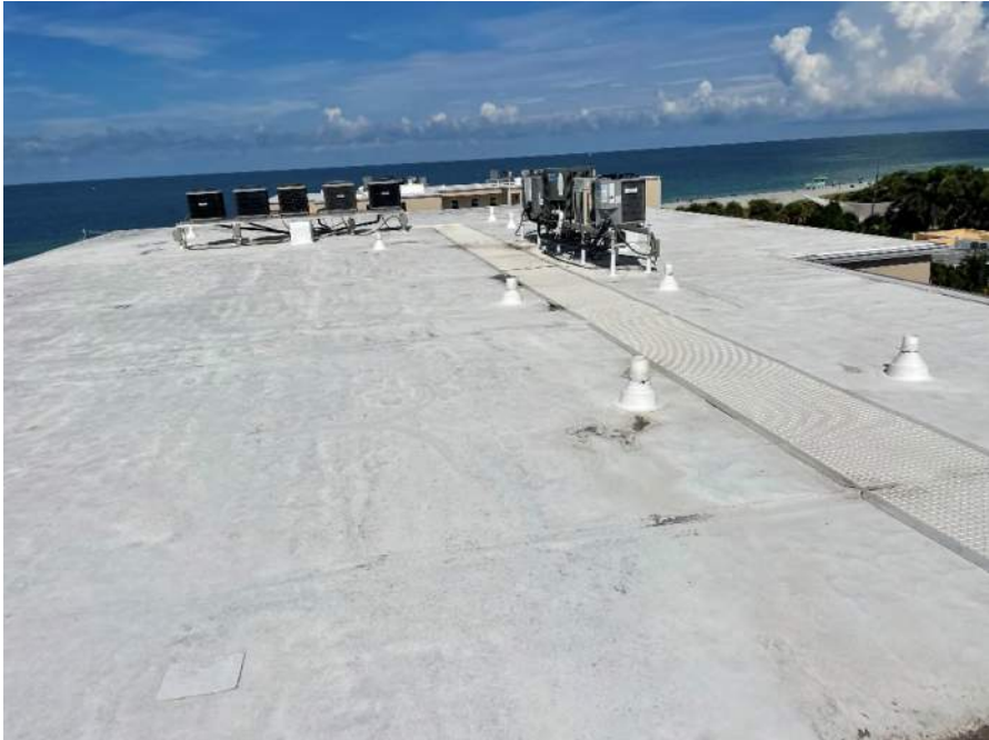
Figure 24 Flat roofing at Grenada Building
