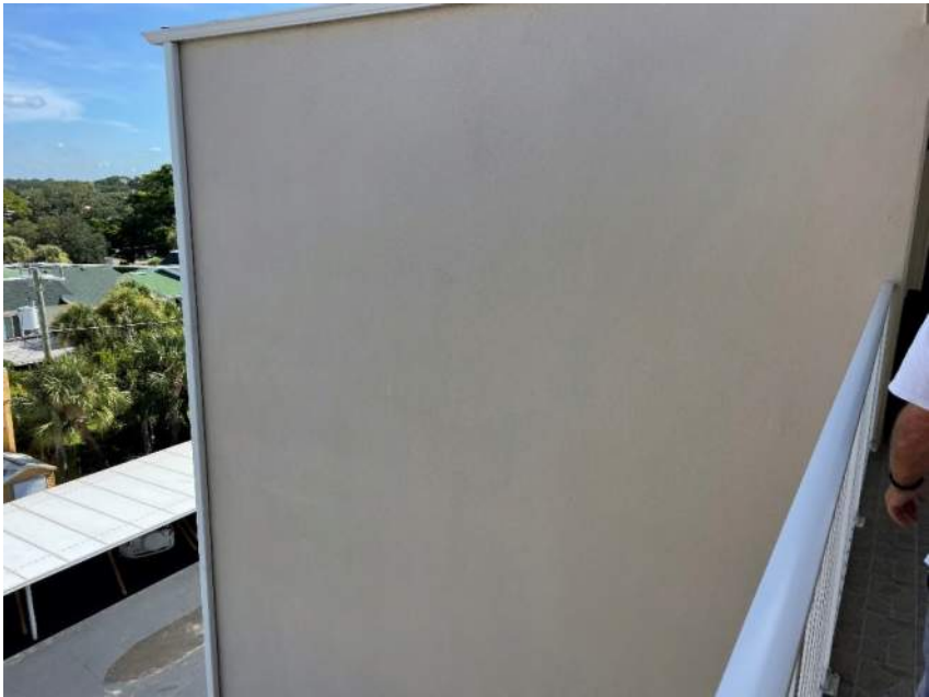
Figure 26. Paint at Golden Strand typical and in good condition
