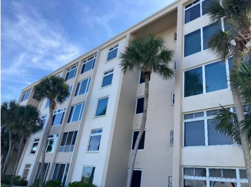
Figure 7 Typical columns on exterior face
