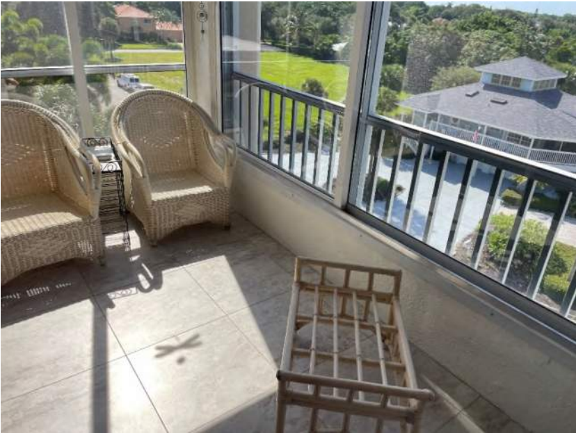
Figure 32 Typical Tiled Balcony at Golden Strand with railing enclosure on outside
