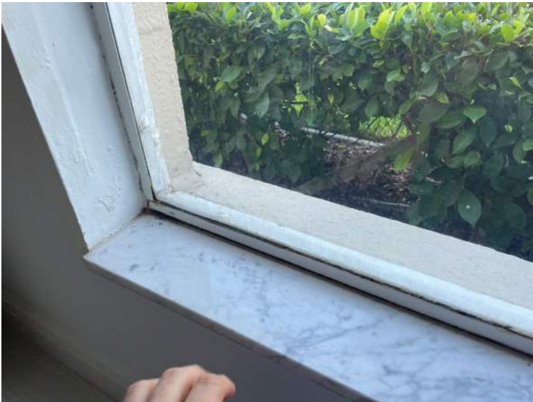
Figure 28 Example of window conditions from the interior
