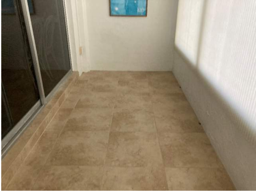
Figure 31 Typical Balcony at Golden Strand
