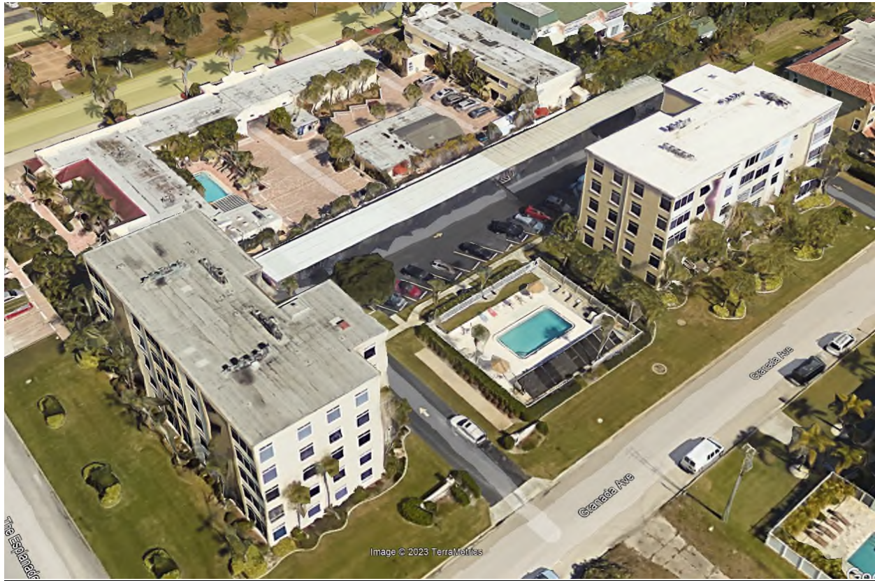
Figure 1 Esplanade Building (left) and Granada Building (right)
