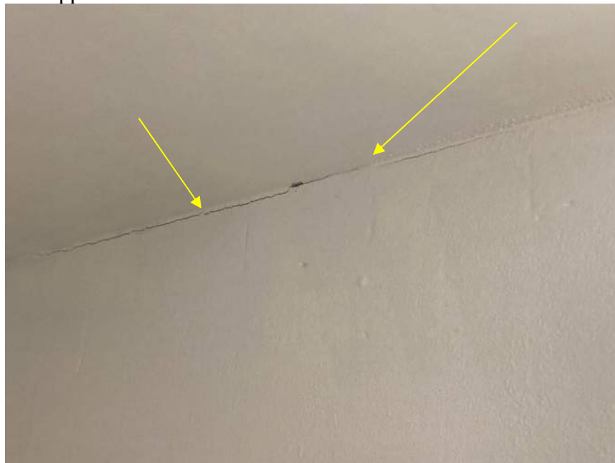
Figure 16 Typical finecracks
