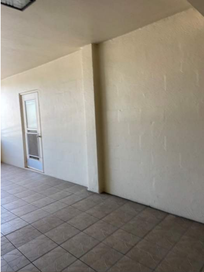
Figure 3 CMU construction in between columns
