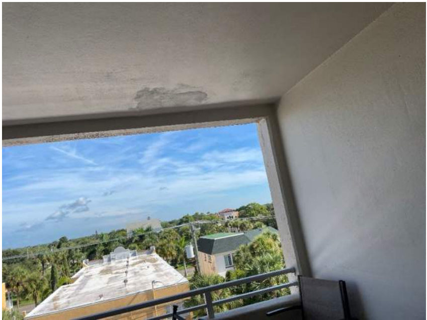
Figure 27. stucco previous repair noted
