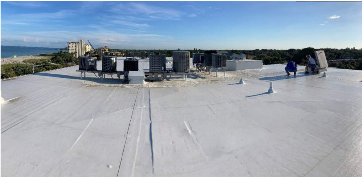
Figure 25 Flat roofing at Esplanade Building
